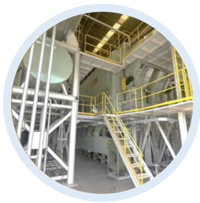
Biomass Boiler size 15 Ton/hour
